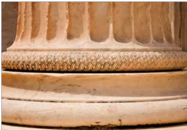
Figure 1 Triple guilloché band on the column base at the Parthenon on the Acropolis
